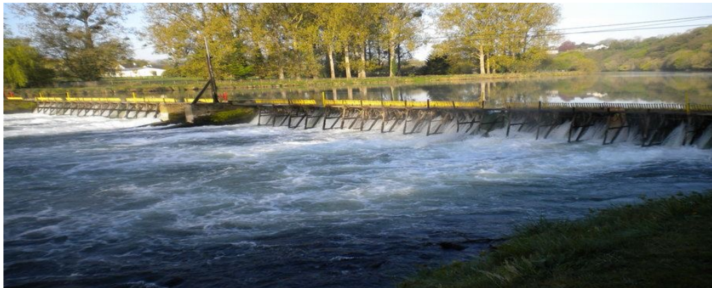
VNF Dams renovation, France
