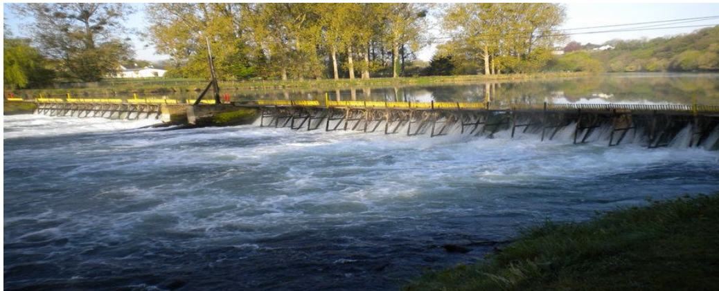
VNF Dams renovation, France
